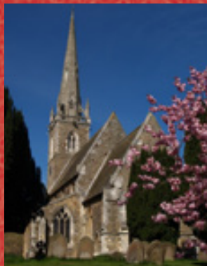
All Saints, Newton-on-Ouse Roof repairs
