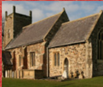
St Margaret's, Long Riston Bell tower repairs
