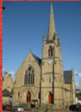
Highfield Trinity, Sheffield Stonework repairs
