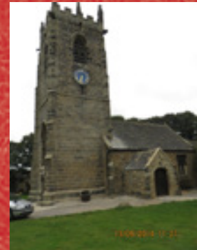
St Michael & All Angels Emley. Roof repairs
