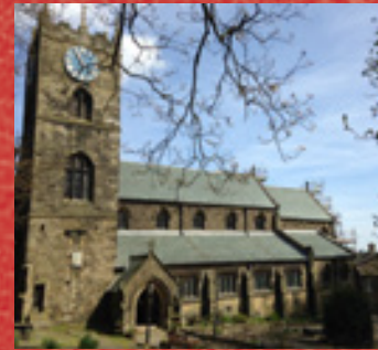
St Michael & All Angels, Haworth Roof Repairs
