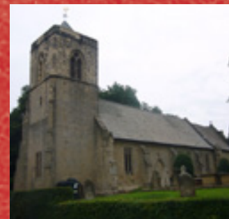
St Mary's, Little Driffield Tower repairs
